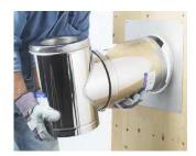
5- You can now install the wall support. Simply slide the wall support up to the tee, ensuring that the adapter on the support engages with the female coupler on the bottom of the tee. When the wall support is level and properly positioned, you can use lag bolts to secure it into the wall studs. TO complete the installation, install an insulated tee plug below the wall support.
